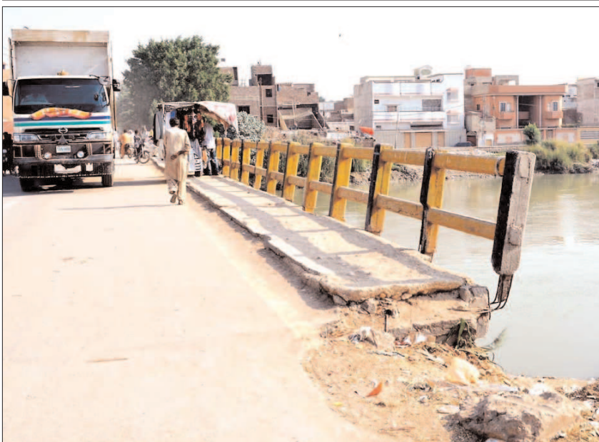
HYDERABAD: A view of damaged safety grills at Kali Mori Bridge, which needs attention of authorities concerned.
