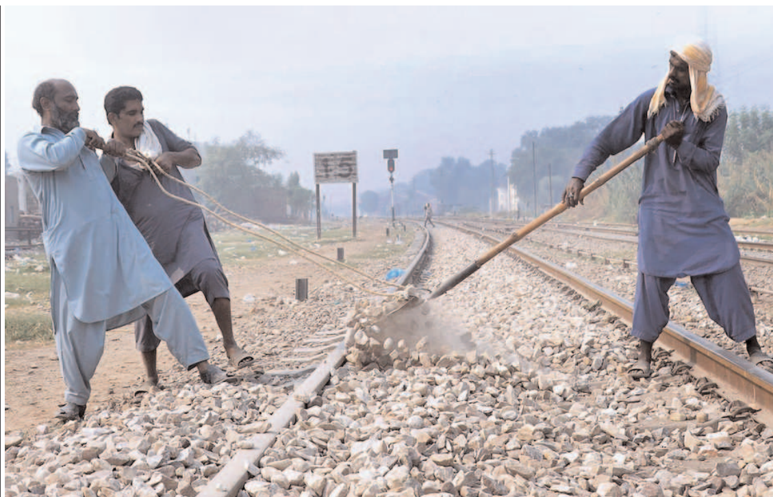
MULTAN: Railway workers busy laying stones around railway tracks during maintenance work near Timber Market.
