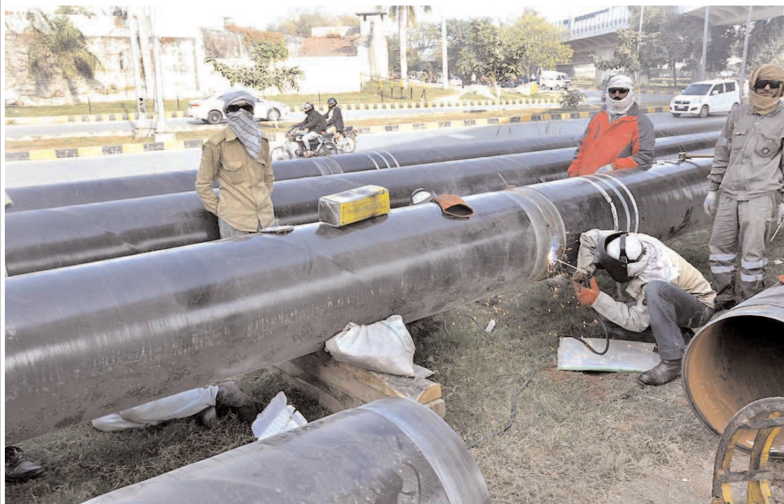
ISLAMABAD: Labourers busy in welding sui gas pipes for laying near Srinagar Highway in Federal Capital.
