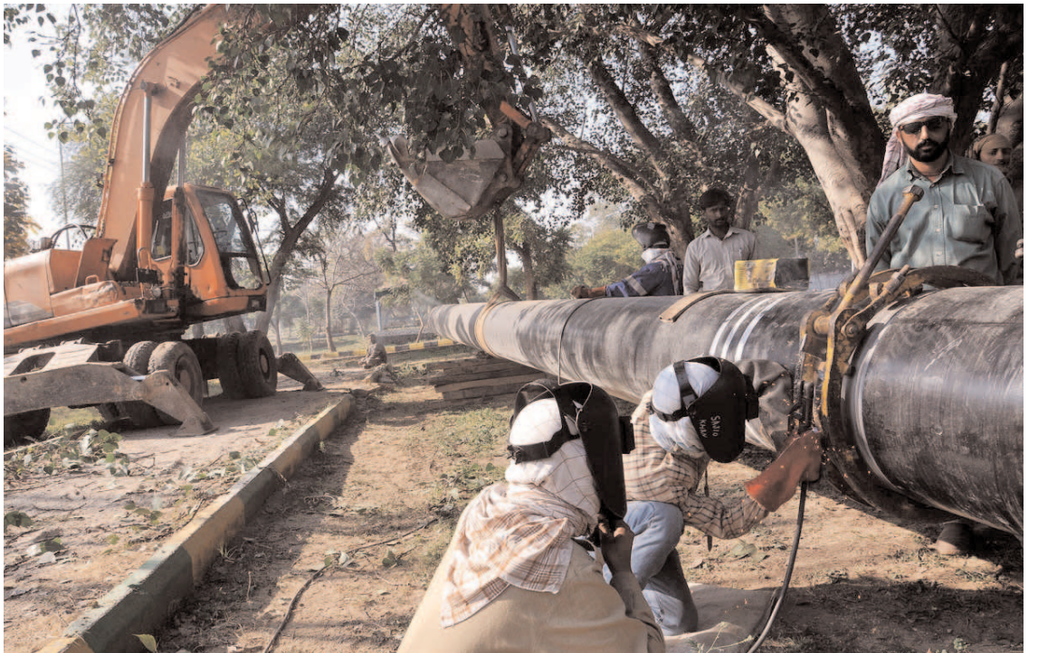
ISLAMABAD: SNGL staffers busy welding gas pipeline during installation at G-7 area in the Federal Capital.
