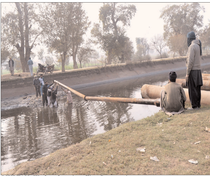
MULTAN: Workers busy installing Sewage pipes.
