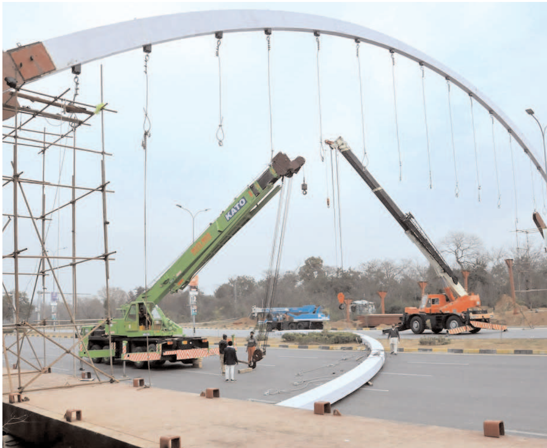
ISLAMABAD: CDA workers busy installing pedestrian bridge with the help of cranes at Srinagar Highway in the Federal Capital. —APP Photo
