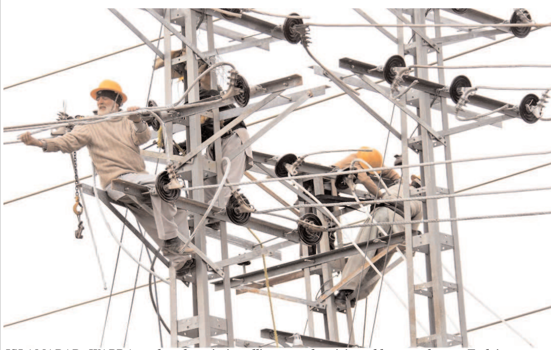
ISLAMABAD: WAPDA workers busy in installing new electricity cables on pylons at Tarlai.
