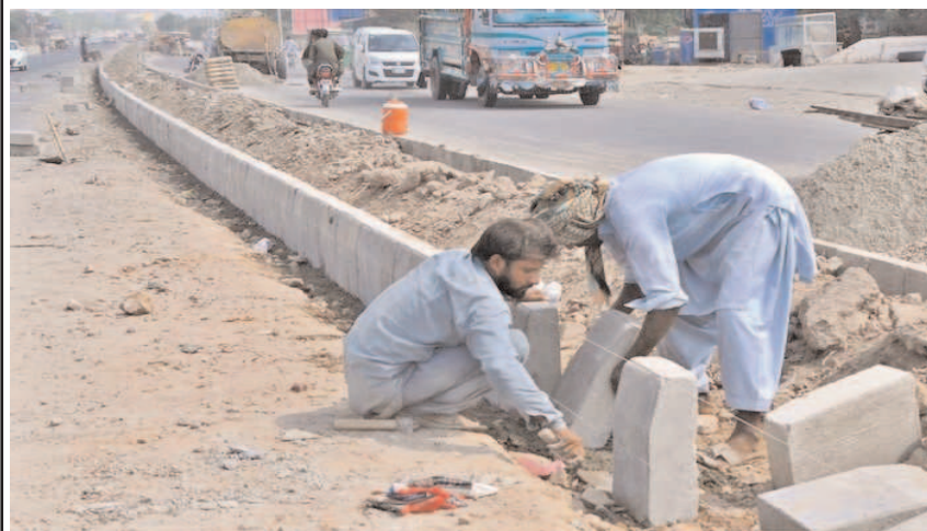
MULTAN: Laborers are busy fixing the cement blocks at the center path of the newly constructed Head Muhammad Wala Road.
