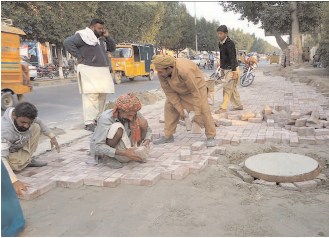
BAHAWALPUR: Laborers busy fixing tuff tiles on footpath.
